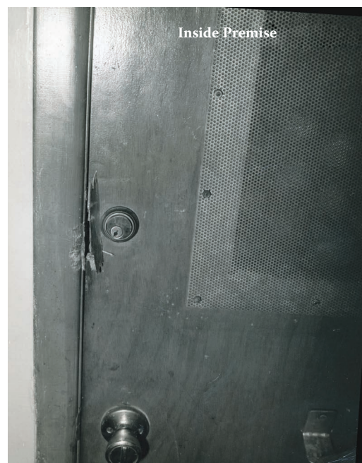
Figure 7.30 Inside of the basement's rear door showing damage on door and door jamb next to lock cylinder.
